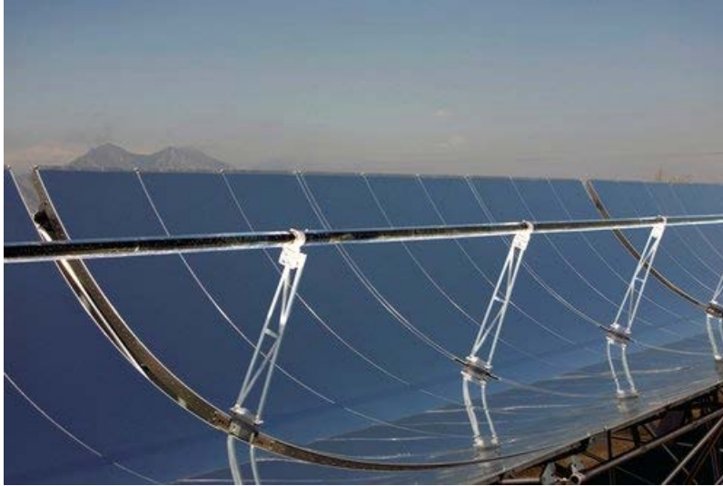
Figure A13. Parabolic trough collector and receiver tube. Photo from NREL 16604
