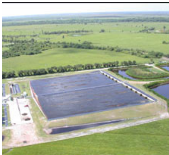
Figure A26. Algal Turf Scrubber® S-154 pilot plant in Central Florida. 95
