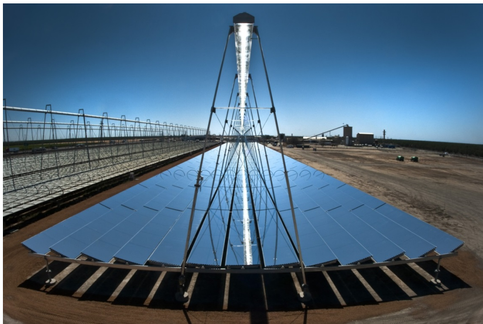
Figure A15. Linear Fresnel system made by Areva. Photo from NREL
