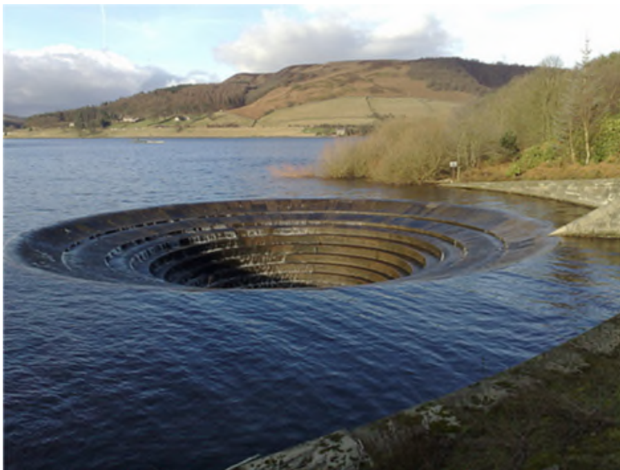
Figure 27 Photo of a Typical Bellmouth Spillway
